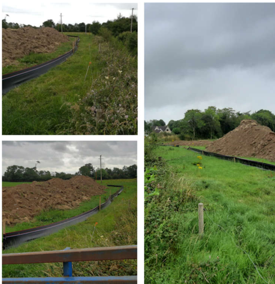
Plate 3-5 Examples of Silt fences
