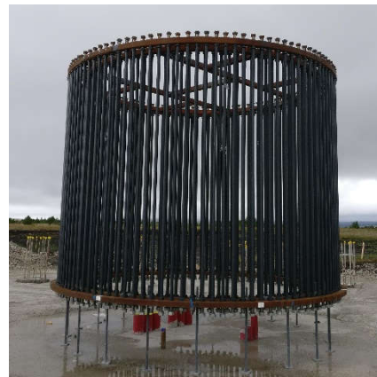
Plate 3-2: Turbine Anchor Cage with Adjustment Feet
