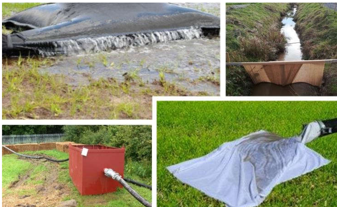
Plate 3-4 Examples of Proprietary Silt Control Measures
