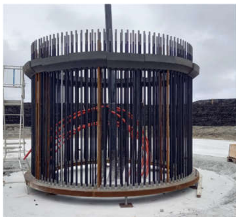
Plate 3-1: Levelled Turbine Anchor Cage
