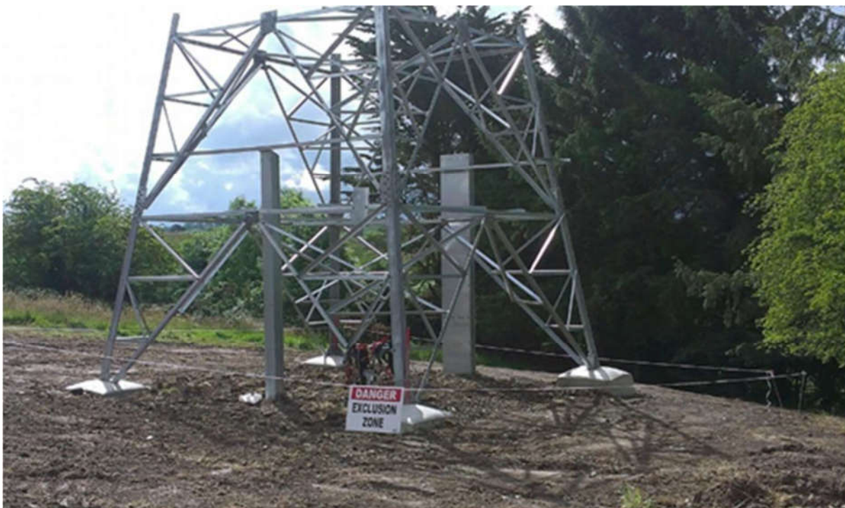
Plate 3-9 Steel lattice tower foundation complete
