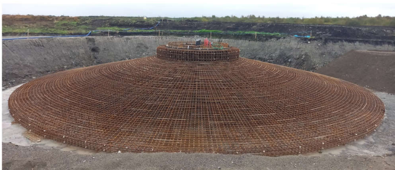
Plate 3-3: Completed Turbine Base Cage
