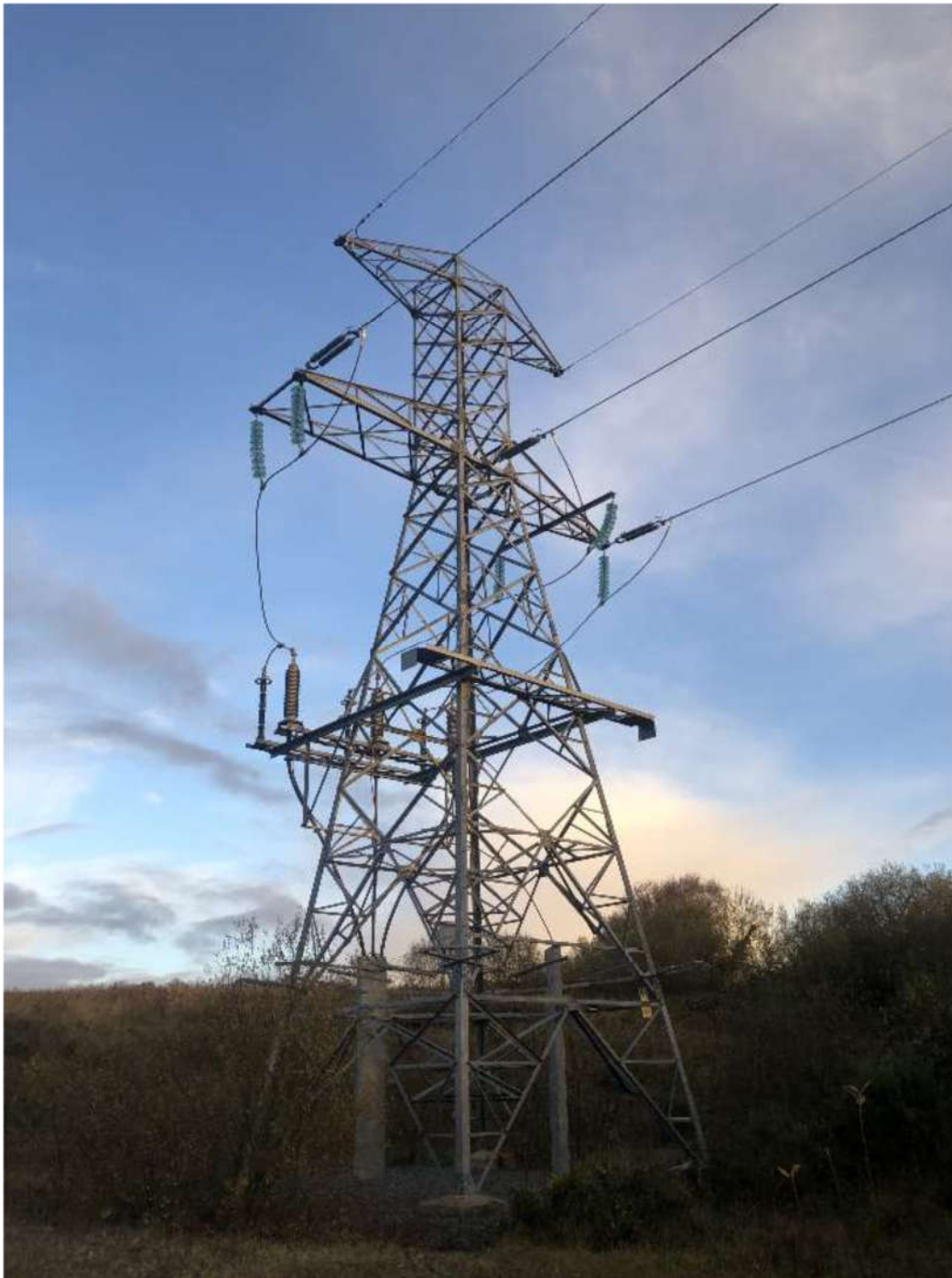
Plate 3-10 Typical Completed End Mast Tower
